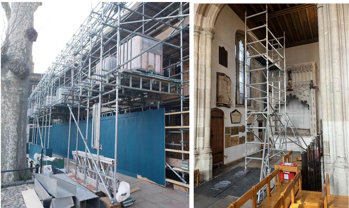
External scaffold build and temporary scaffolding for the monument survey.
